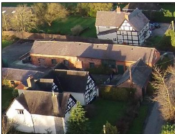
Farmstead complex at Tilley Manor
