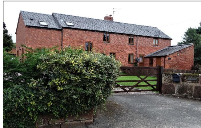
Tilley Barn, formerly part of Brook Farm
